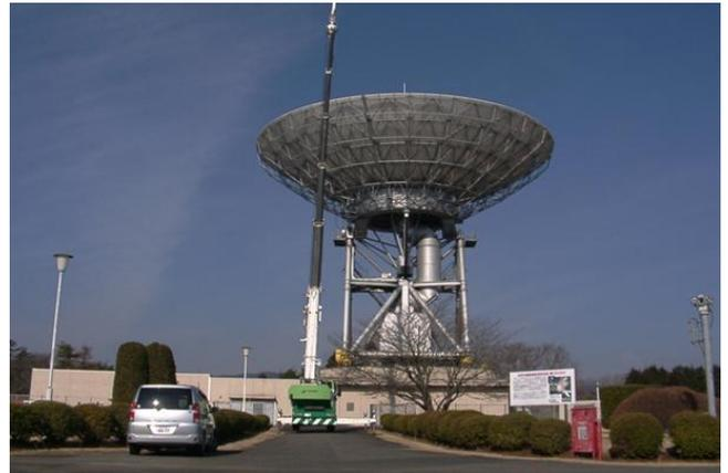
Fig.14 Feed installation
