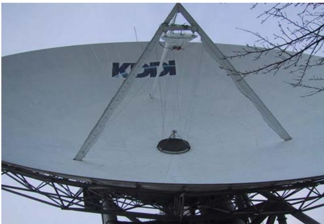
Fig. 16 KDDI antenna equipped with 2m, 70cm and 23cm feeds.
